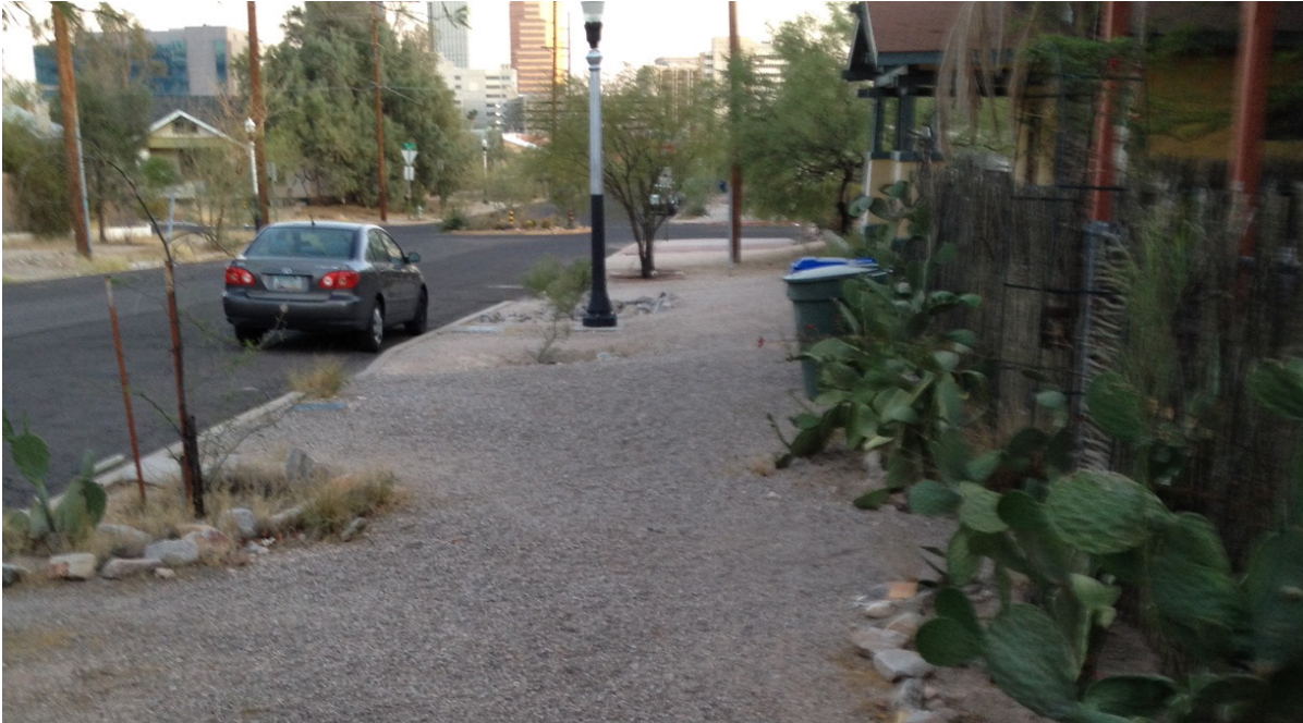
Gravel in walkway at 721 N 9th Ave makes walking or pushing stroller difficult. Pathway is clear. -Brad Lancaster
