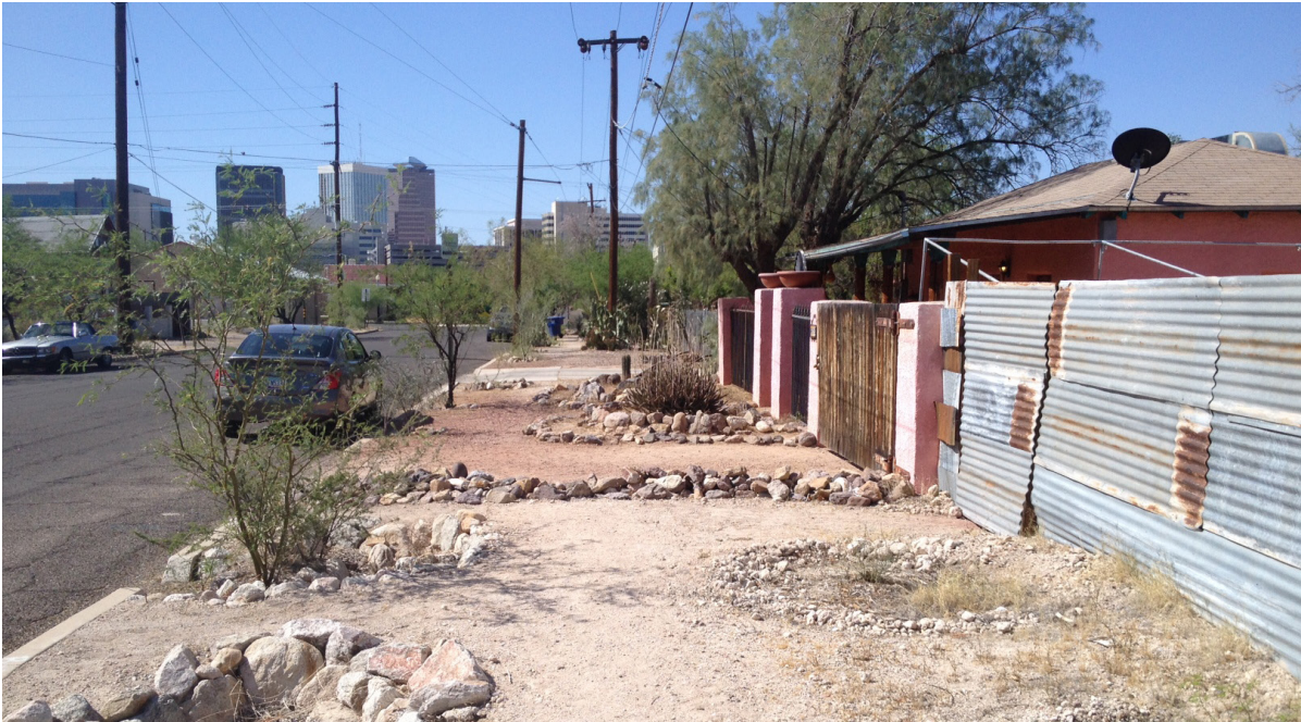
At 631 N. 9th Ave, rocks block path. Rocks along path make it too narrow - only four feet wide.
