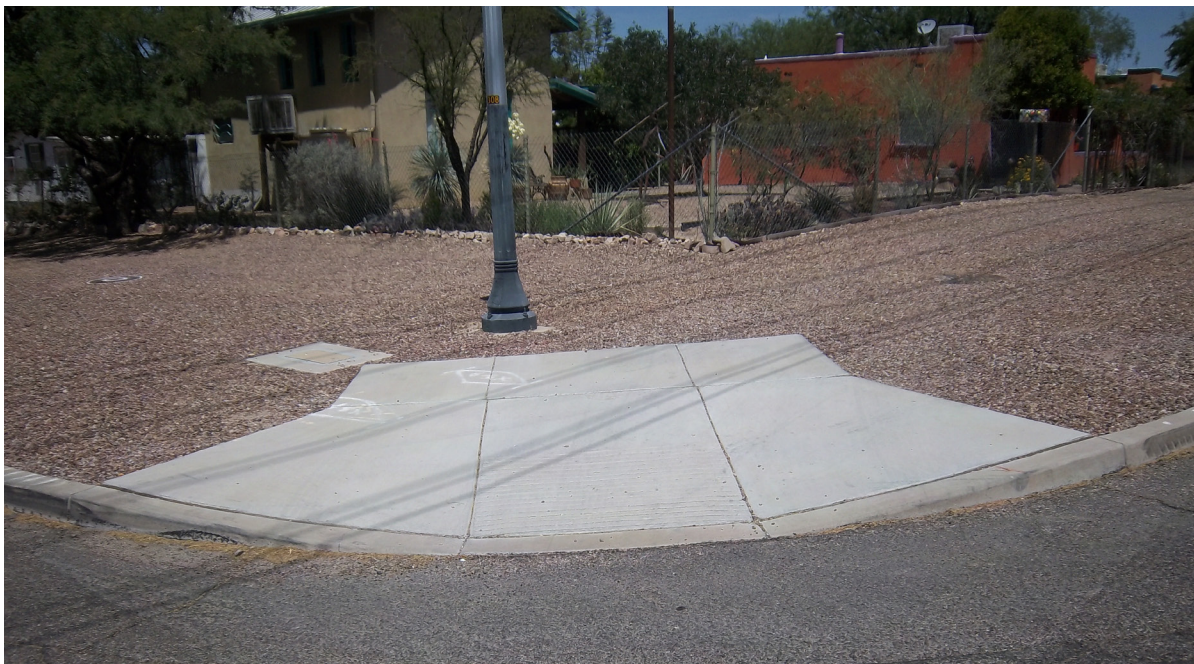
Handicapped access to nowhere due to loose gravel at 11th Ave. and 2nd Street. Pathway is clear.
