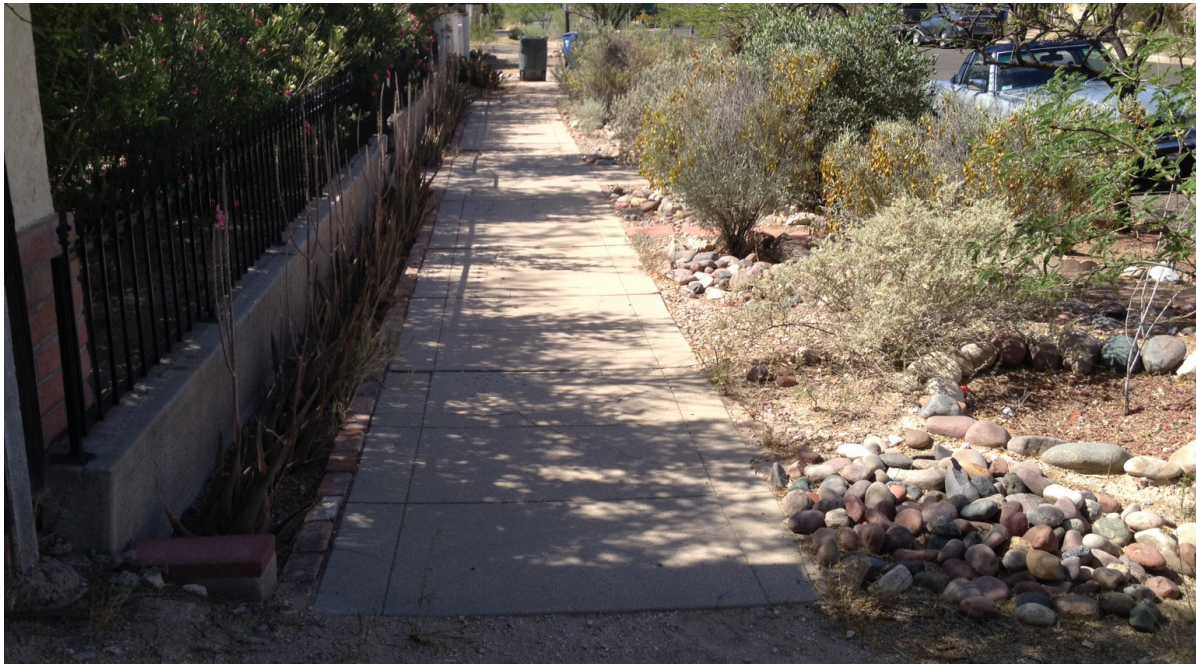
Only sidewalk is in front of 628 N 9th Avenue (historic home). Nice clear and wide. Over five feet wide. But it needs repair. Neighbors garbage cans at 618 N 9th Ave somewhat block path on south end.
