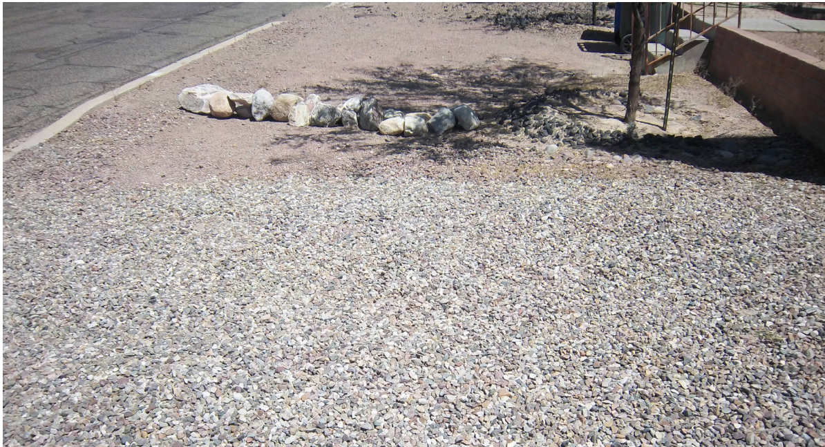
Impassable sidewalk on 11th Ave south of University Blvd. due to loose gravel and rock barrier.
